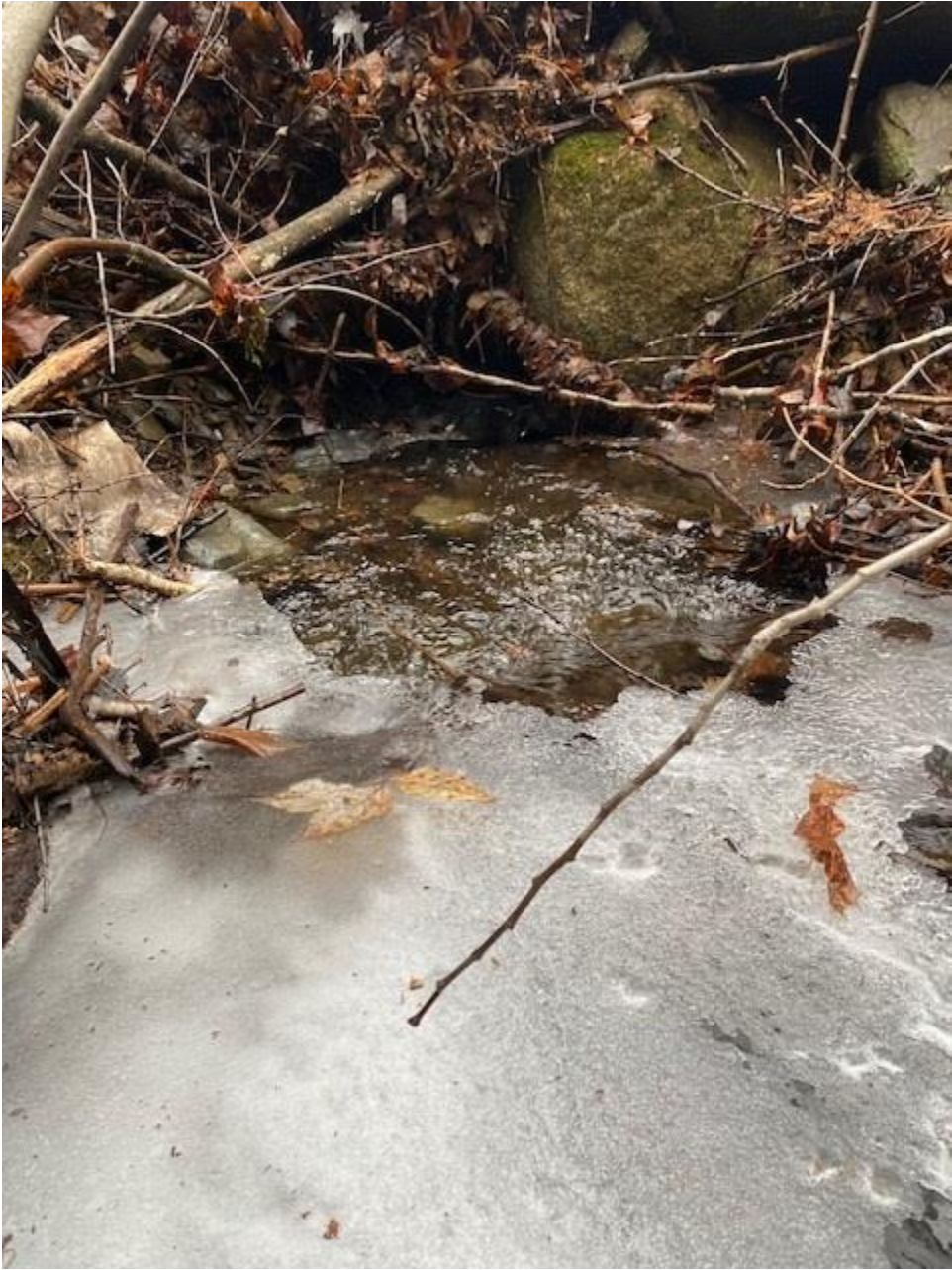
Hudson Road Culvert - Left
