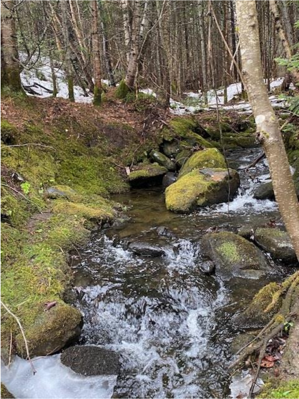
Hudson Road – Bolter Brook Left going into Culvert
