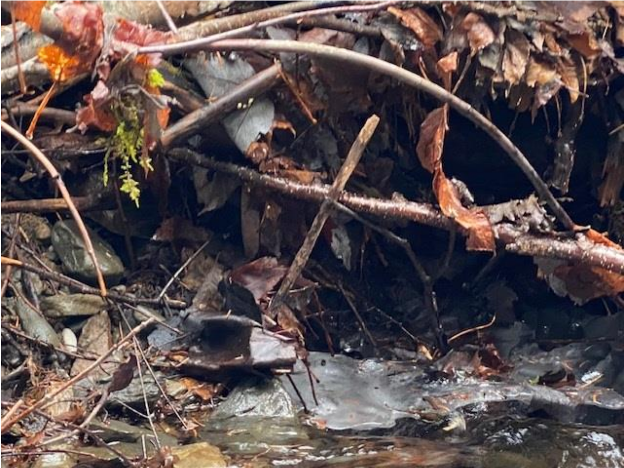
Hudson Road Culvert Left
