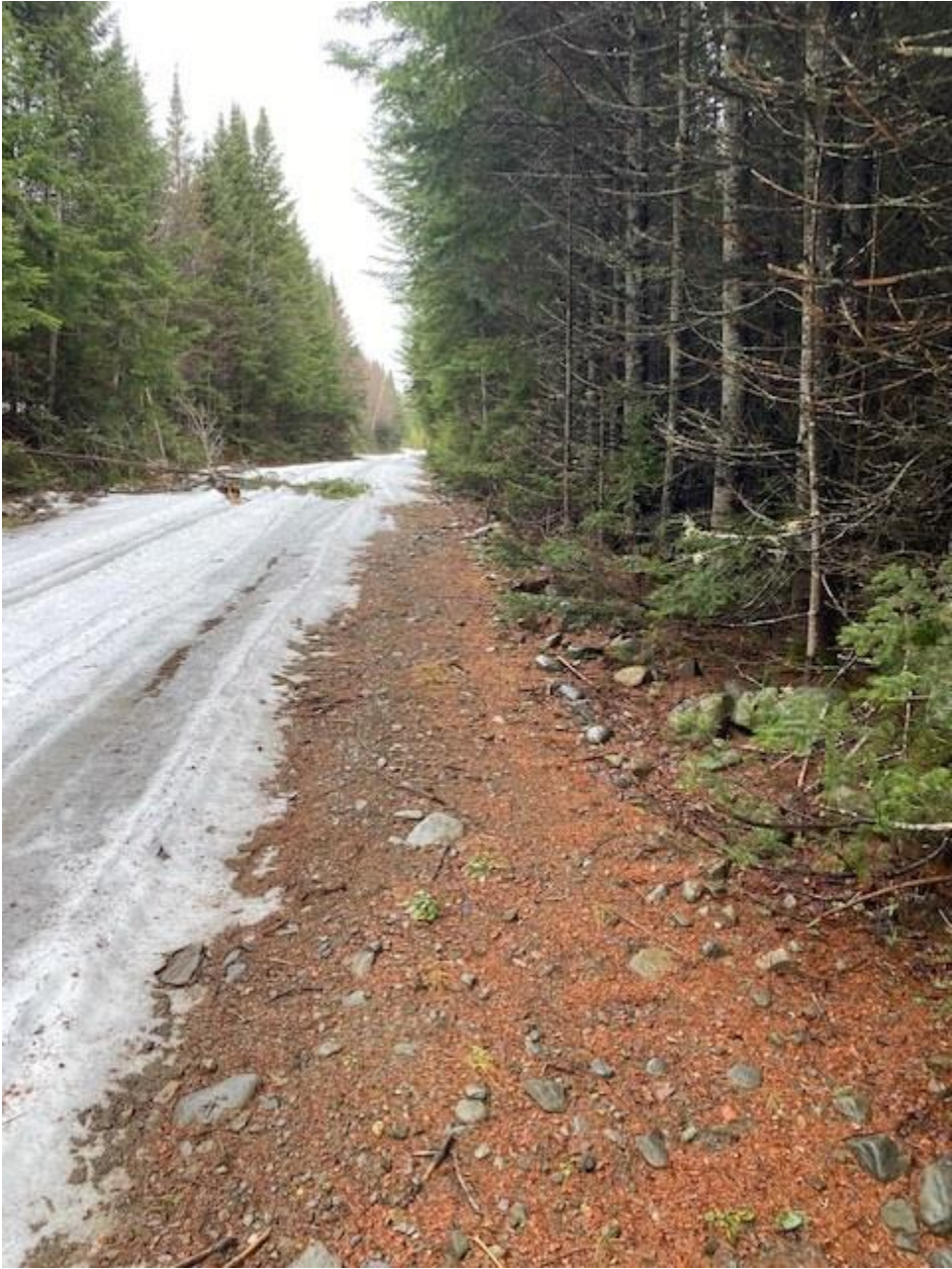
Hudson Road Right Ditch
