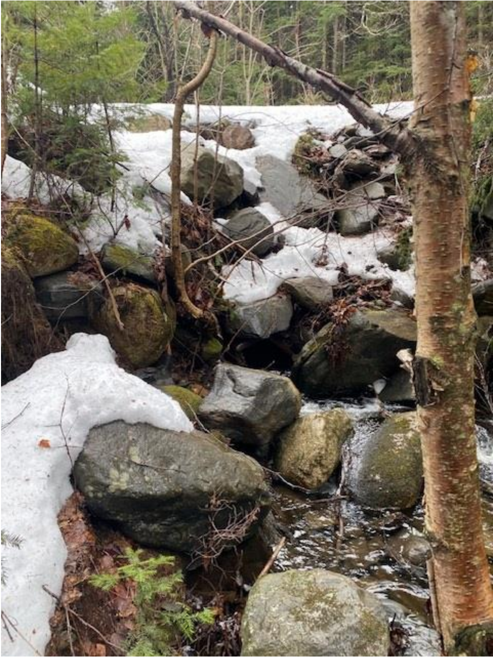
Hudson Road – Culvert Right
