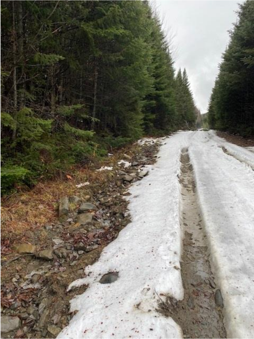
Hudson Road Left Ditch
